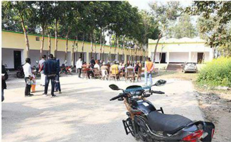
Main Building Varamda Right Side View
