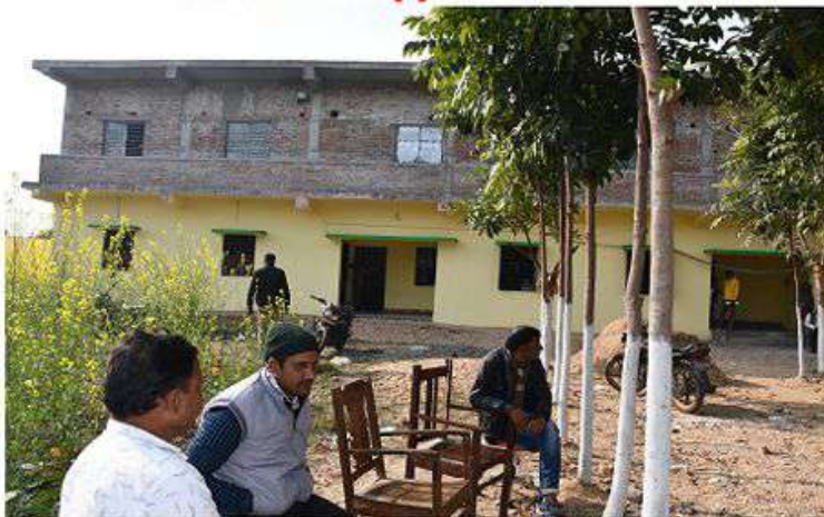
West Side Upper Hall View
