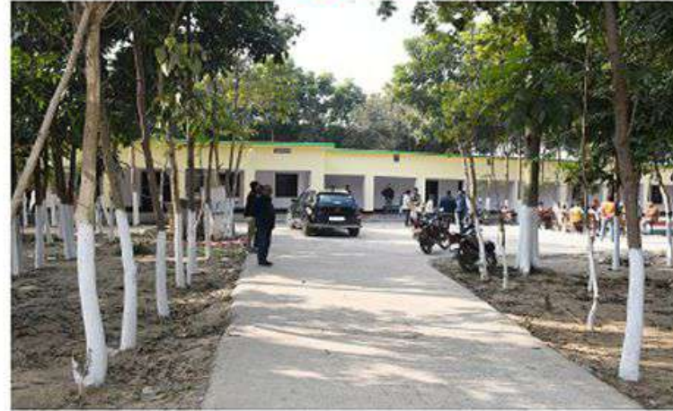
Main Building Front Side View
